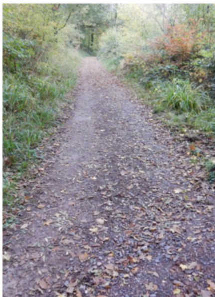
The path after repair
