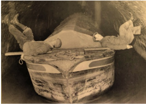
'Legging' a Canal Barge through the tunnel
