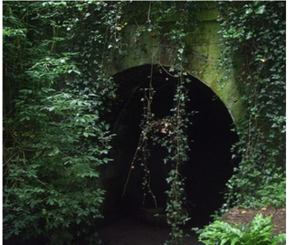
North Entrance to Crimson Hill Tunnel
