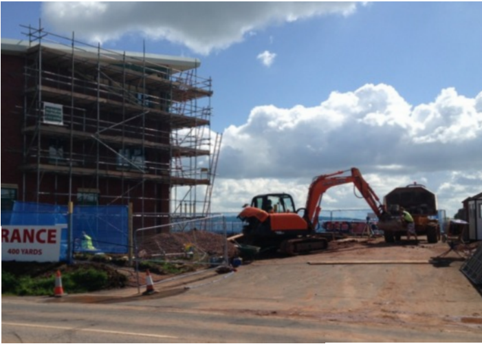
The first of the scaffolding
