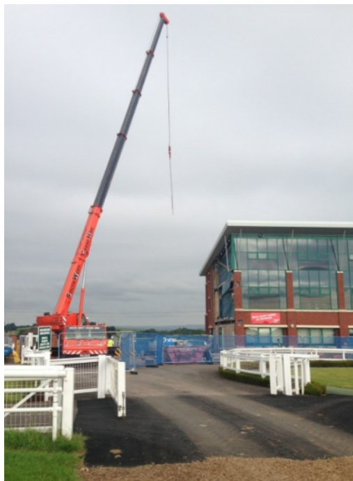
The contractors arrive
